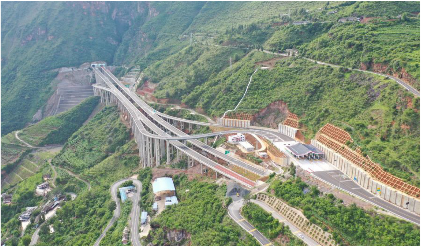
The Jin'an interchange is one of many components of the Yunnan Huali Expressway Project in China, which won Best Road/Highway. Photo courtesy CCCC
